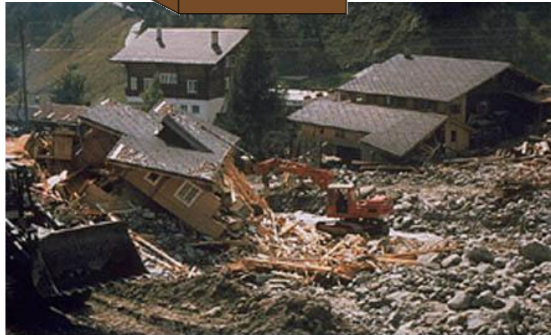
Houses undermined by melting Permafrost
